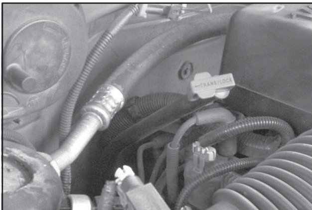
ILLUSTRATION 3: A/C ACCUMULATION LINE DRIPS WATER ONTO CAP
